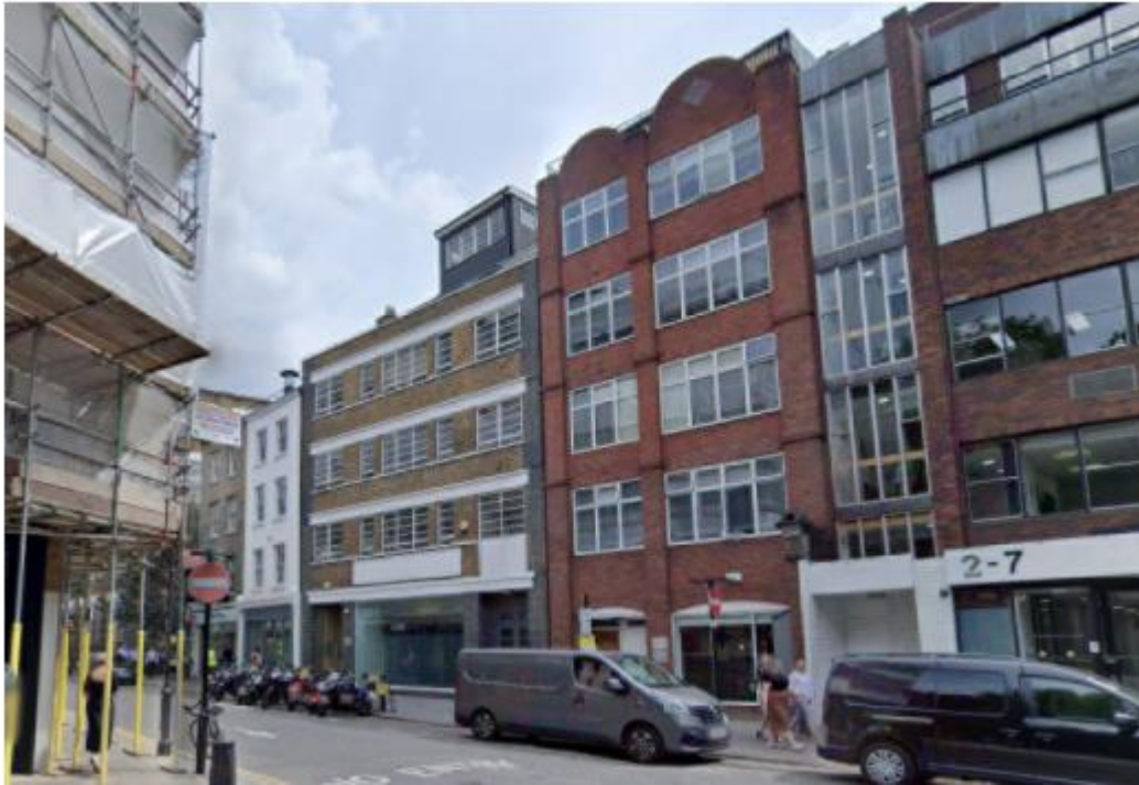
Image 4: View east from the corner of Sekforde Street and Clerkenwell Green
